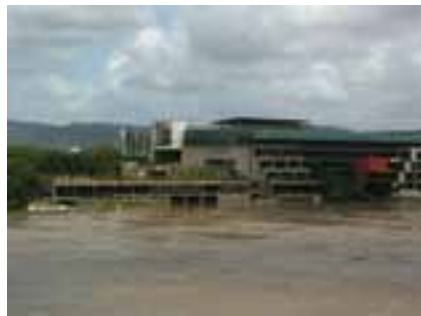
State Library of Queensland and The Edge inundated
